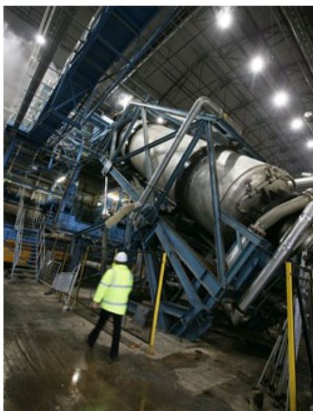
Stereecycle has stopped processing waste at its Rotherham facility
