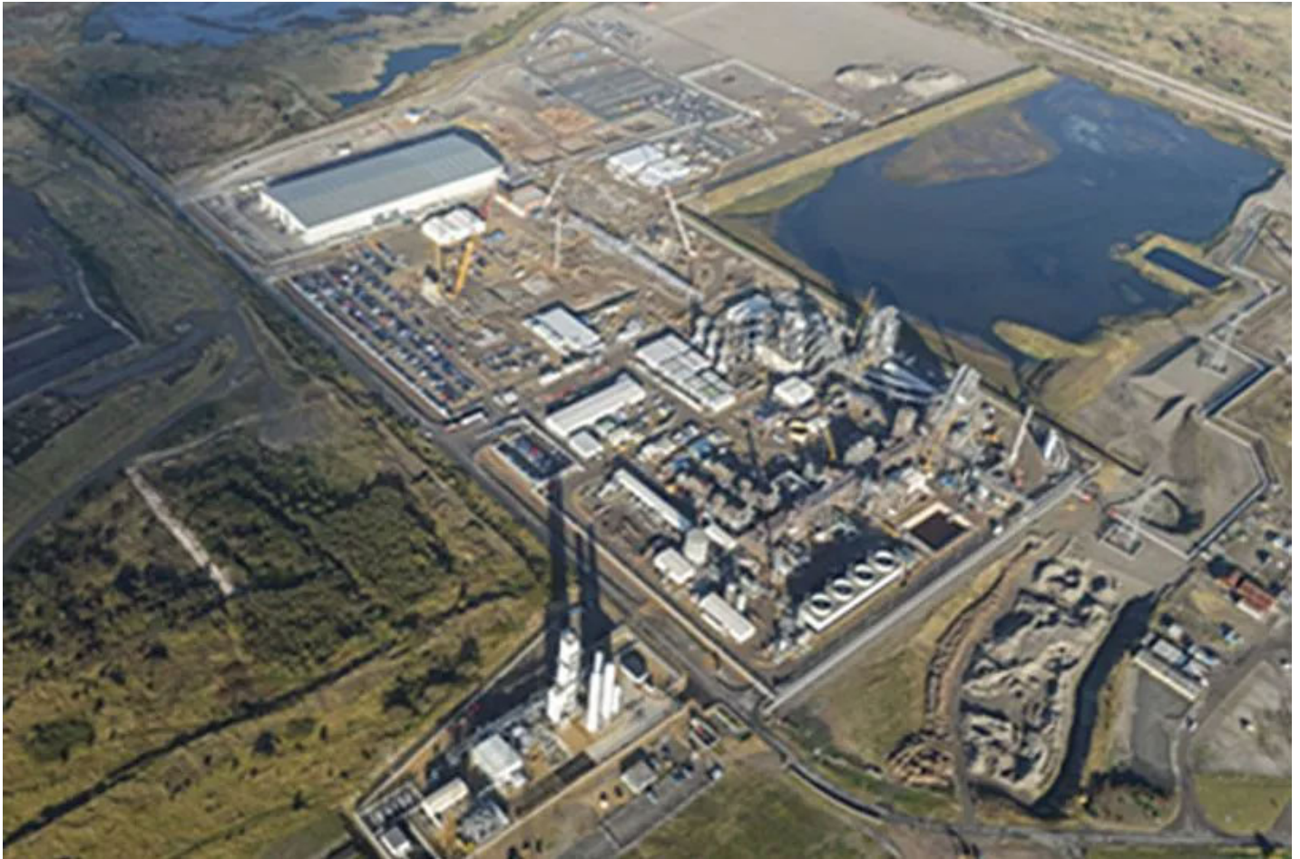
Locator of Air Products' Tees Valley Renewable Energy Facilities
